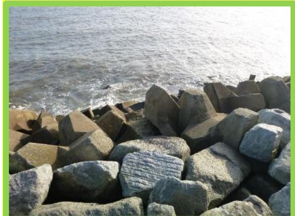
*Example of locally cracking and movement of Accropode units, but otherwise revetment in good condition (/1202C02)*
