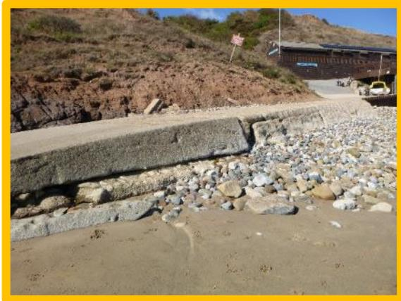
Evidence of voids forming beneath boatyard ramp (/1601C03)
