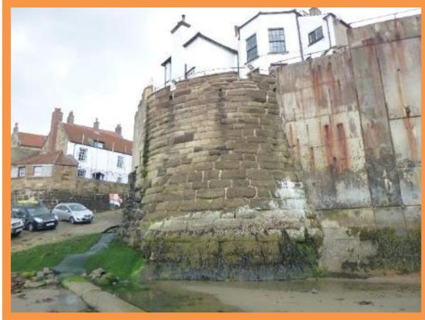
*Blockwork wall in poor condition fronting the Bay Hotel (/1003C04)*
