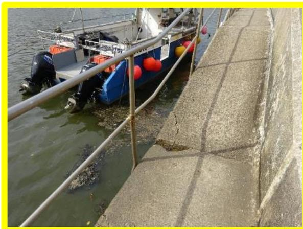
*2020 - Local damage. Cracking and loose concrete to crest of South Breakwater (/0403C03)*
