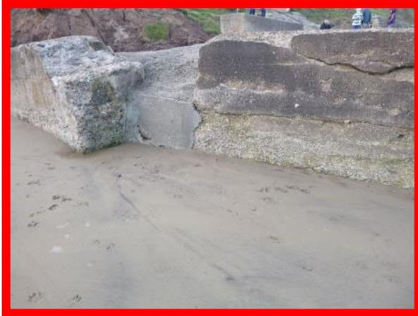
Concrete skim repair has filled voids and cracks (/1402C06)
