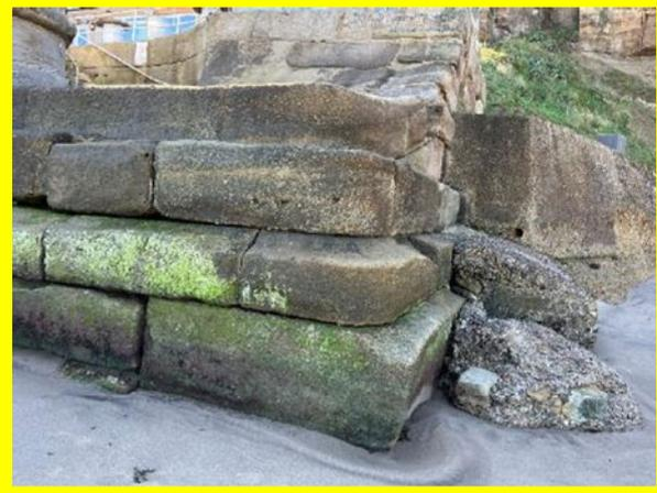
Open joints in wing wall to access steps (D0802C12)
