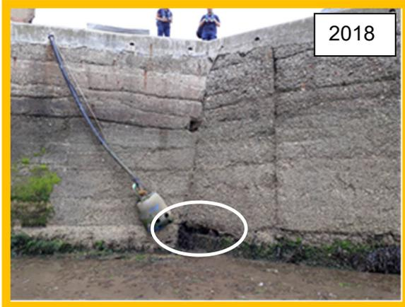
*2018: Void at toe in south face of West Pier wall and damaged conduit (/1301C07)*
