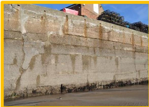
*Longitudinal cold joints in south face of West Pier wall (/1301C07)*
