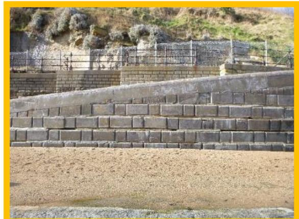
*Seawall in overall poor condition Cracks to bastion throughout. Mortar missing between blockwork in lower wall. (/1304C02)*
