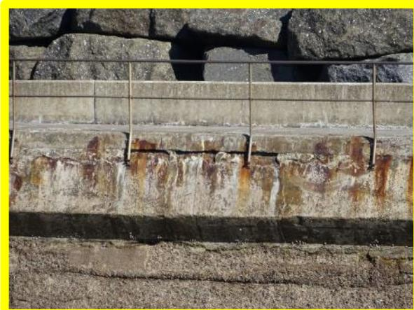
*Rust staining and opening of construction joint on inside face of structure (/0402C01)*
