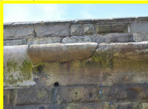
*One remaining section of damage to the bullnose wave deflector (/1301C27)*
