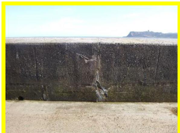
*Cracking in crest wall (/1201C02)*
