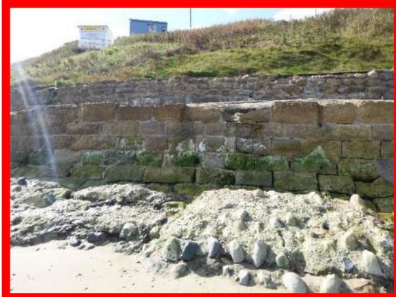
Missing mortar and damaged blockwork (/1402C04)
