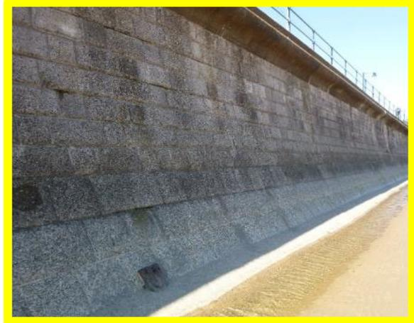
Evidence of ongoing abrasion on wall face. Low beach levels expose concrete toe (/1602C08)
