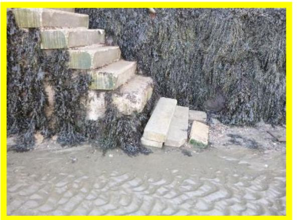
*Access steps at root of East Harbour pier in poor condition. (/1301C01)*
