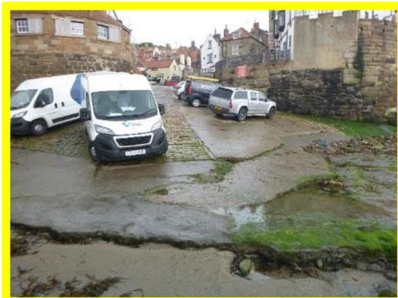
*Slipway in fair condition, but with undercutting at the toe (/1003C05)*
