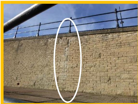
*Original vertical crack in wall above access ramp (/1301C10)*
