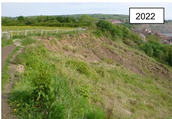
Head scarp of MU17/2 (Partly Active in August 2022)
