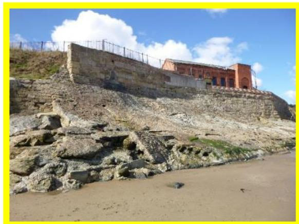
Evidence of voiding and deteriorations of grouted revetment at southern end of defence(/1402C05)
