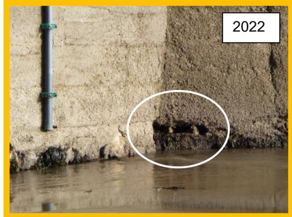
*Spalling and loss of render in south face of West Pier wall. Void remains unchanged (/1301C07)*
