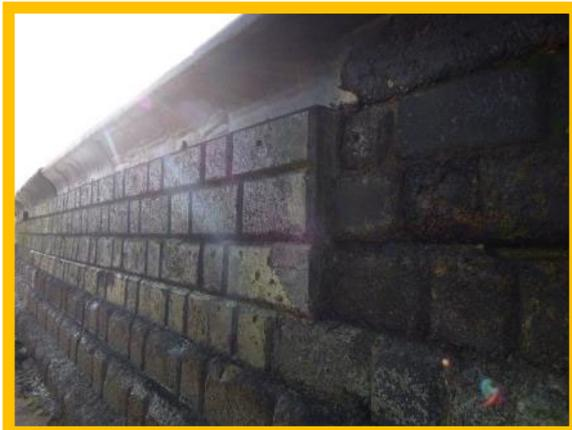
*Repairs to wall face and coping in good condition. Extensive abrasion of adjacent blocks (/1302C02)*
