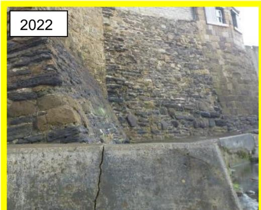
*Typical defects (cracking) on toe apron (/1003C06)*
