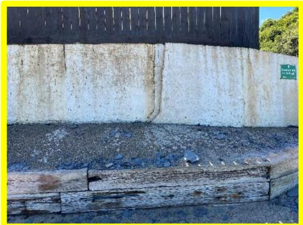
*Crack in concrete wall (/0602C05)*
