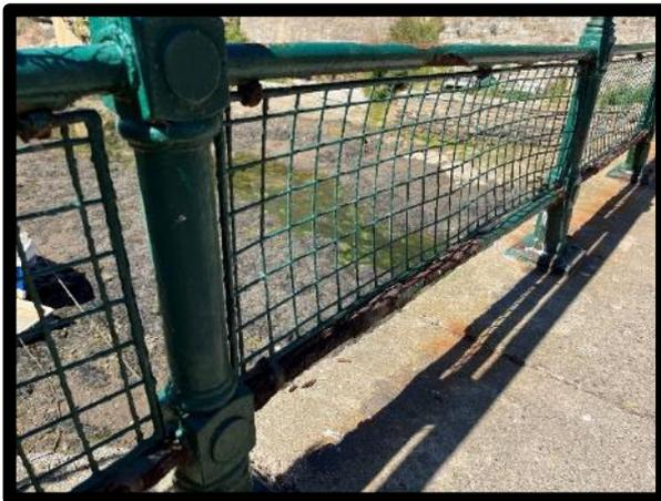
*Footbridge – significant corrosion of bottom rail (no asset ref).*
