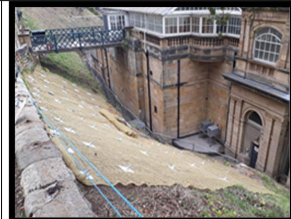
**MU22/2** Soil nail and slope mesh installation behind main Spa building in 2018
