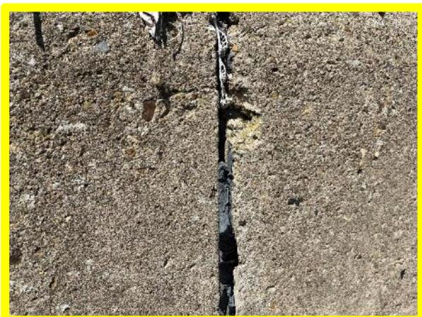
*Brittle/missing sealant in expansion joints (vertical and horizontal). Vegetation growth locally. (/0601C03)*
