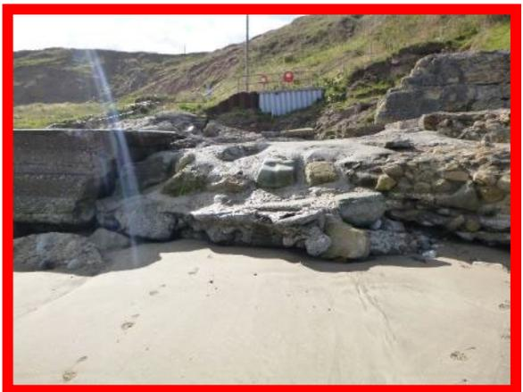
Voiding and undercutting of structure at the interface between (/1402C04) and (/1402C06).
