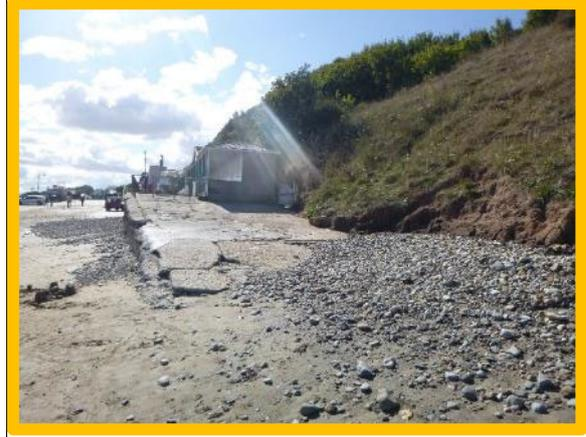
Toe of **MU27/X** showing signs of some localised recession adjacent to the Filey sea defences increasing the risk of outflanking.
