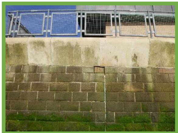
*Dislodged block on new seawall (/1301C08)*
