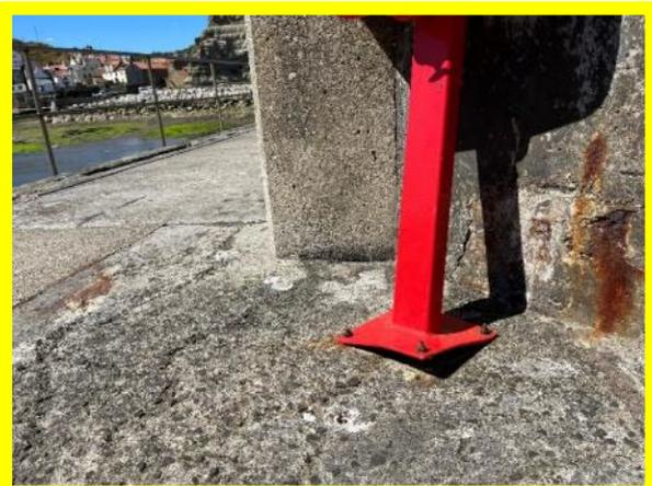
*Damage to base fixings of life-ring mount (/0402C01).*
