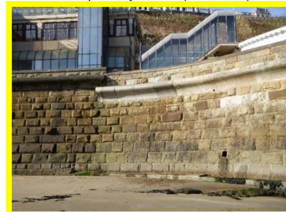
*Previous repairs to the bullnose wave deflector in good condition (/1301C28)*
