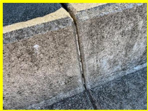
*Brittle/missing flexible sealant from expansion joints (/0403C03)*
