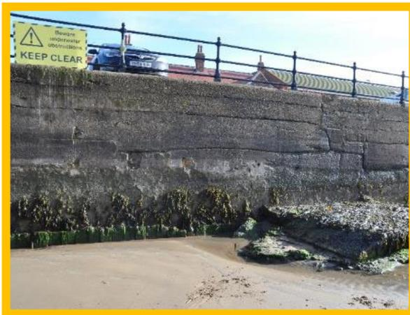
*Large open joints and cracks are evident from along the wall's full extent (/1301C19)*
