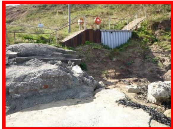
Undermining of footpath beneath 'Lucy's Shack' (/1402C04)
