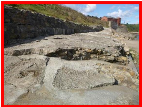
Deck slab repairs in fair condition. (/1402C04)
