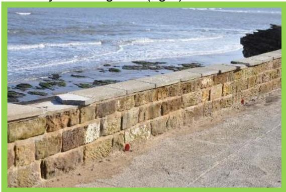
MU22/4 wall coping found to be loose, damaged and missing in places.
