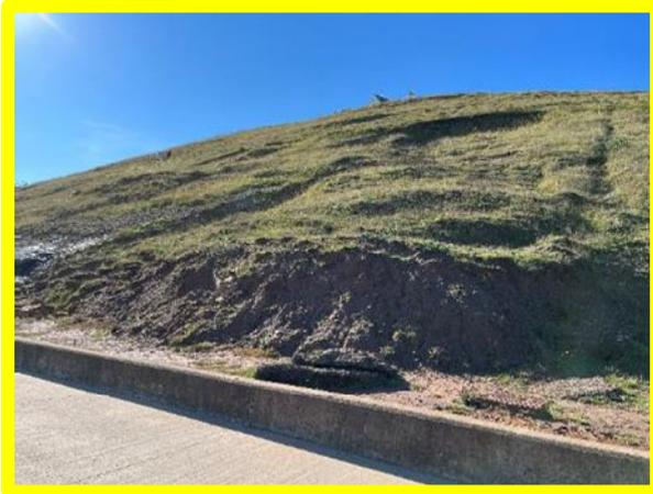
**MU11/1** Evidence of slumping and broken pipe in the lower coastal slopes (Locally Active)
