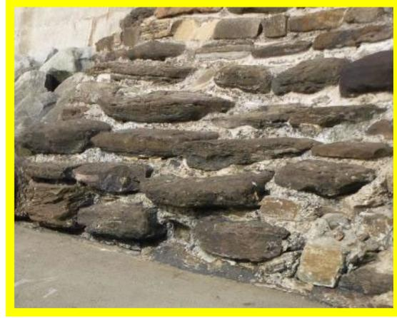
*Typical defects (gaps) on blockwork wall (/1003C06)*
