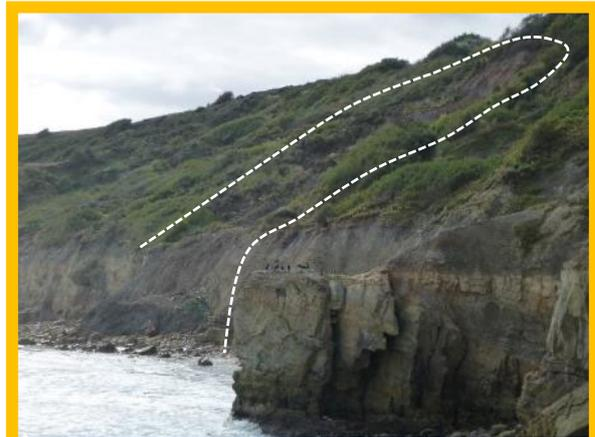
**MU23/A & B** Partially active landslip and debris lobe visible
