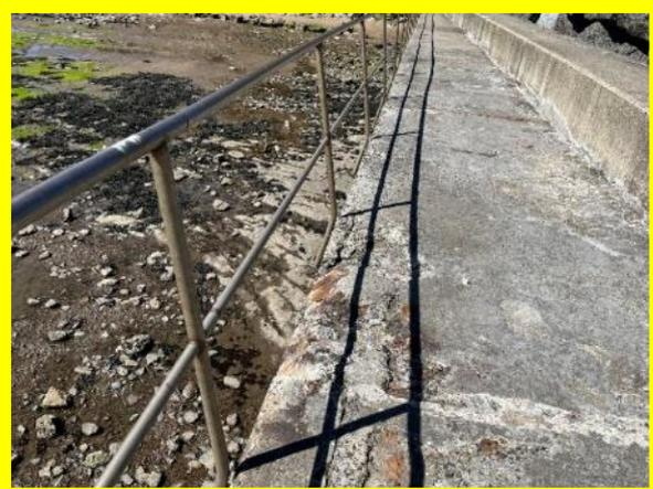
*Abrasion to deck along inside edge of structure (/0402C01)*
