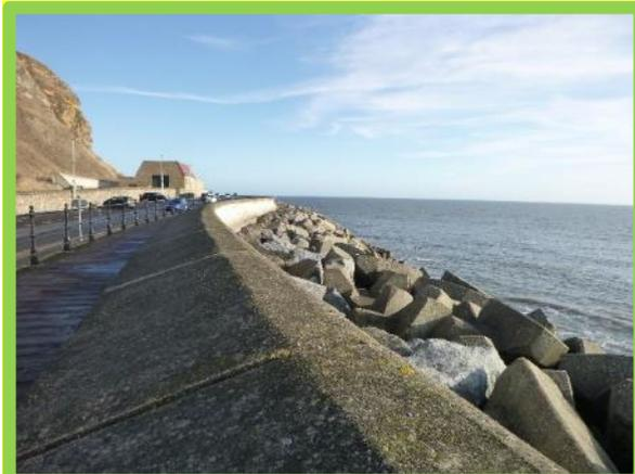
*Accropode revetment with concrete toe piles, rock crest and wave return wall (/1202C02)*
