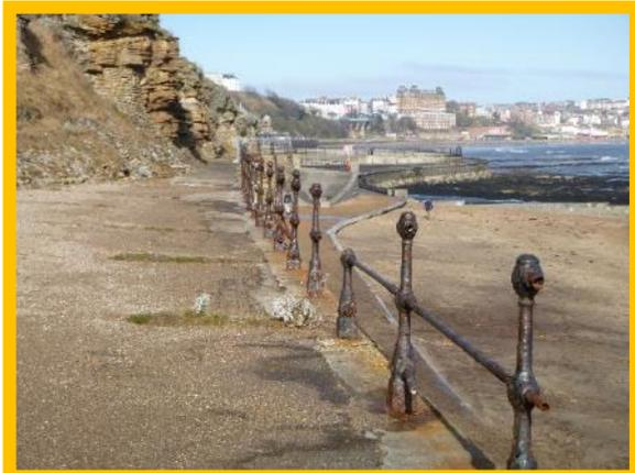
*Upper prom has been fenced off and is in poor condition, heavily abraded and damaged handrail (/1304C02)*
