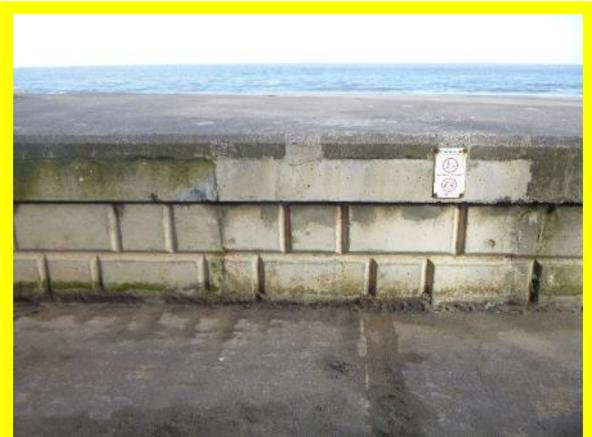
*Vertical crack (seen from rear of crest wall) (/1201C06)*
