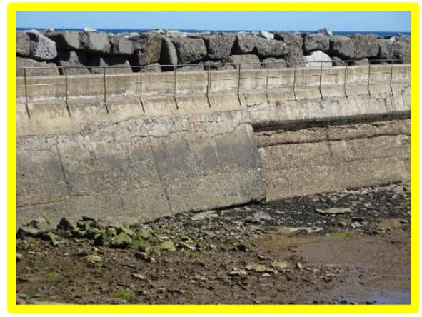
*Detail on potential undercutting (left) and opening of construction joint (right) (/0402C01)*
