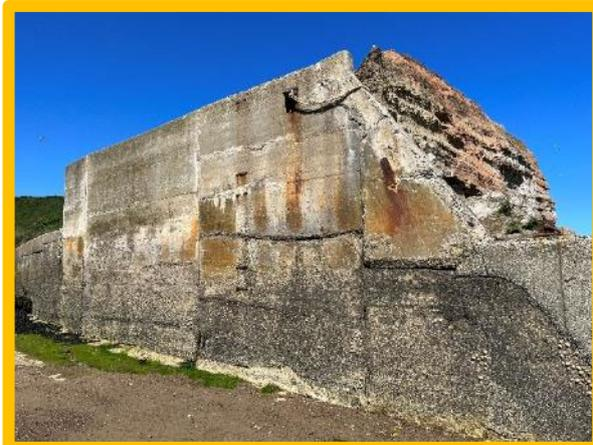
*Cracks and cold joints in concrete seawall to rear of slipway (/0402C03)*
