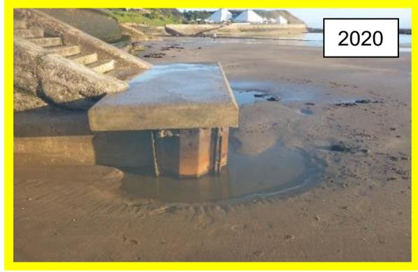
Corroded sheet Piles with minor seaward visible in 2020 (/1201C24)
