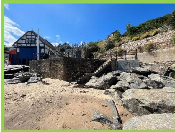
*Break in rock armour fillet at pumping station (/0601C07)*
