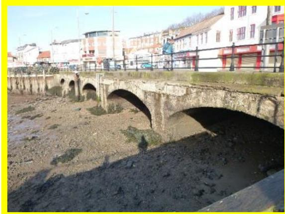
*Some Cracking and missing joints to capping apron to wall south of roundabout opposite arcade. (/1301C05)*
