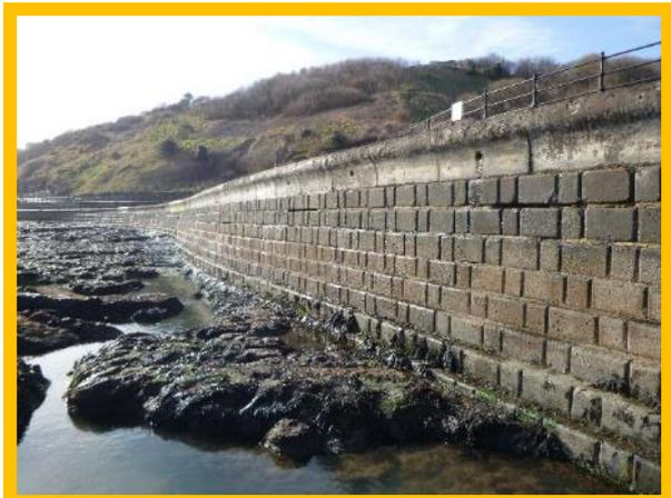
*Previous repairs to wave return coping (/1303C02)*
