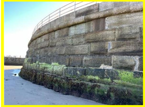
Battery Wall, with some open joints between blocks (D0802C12)
