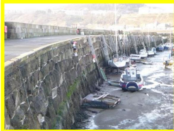
*East Harbour inner pier, historically repaired joints visible (/1301C16)*
