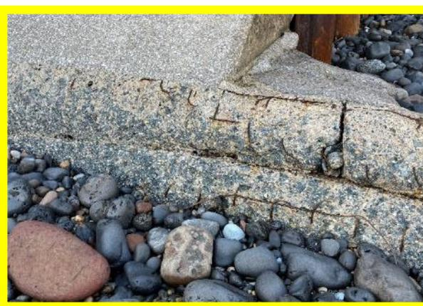
Exposed rebar evident at toe (D0701C02)
