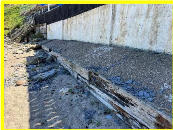
*Rotten/missing timber (permanent formwork for concrete behind) (/0602C05)*
