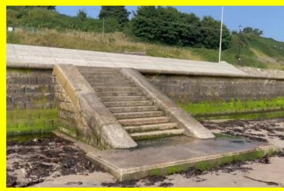
Concrete foundation to access step landing. Sheet piles not visible in 2022 (/1201C24)
