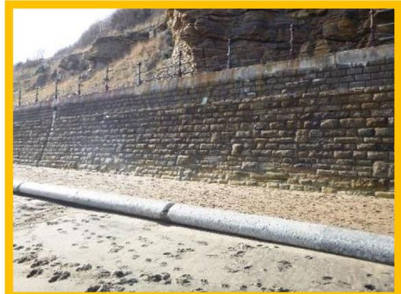
*Missing pointing / open joints and damaged parts of upper and lower capping beam (/1304C02)*
