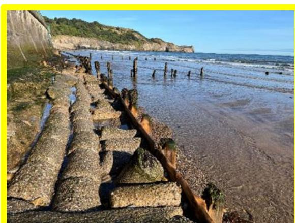
Toe structure formed from concrete-filled barrels (D0702C01)
