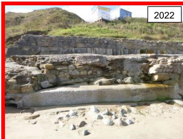
Mass concrete repair to damaged section of wall note undercutting in foreground. (/1402C04)
