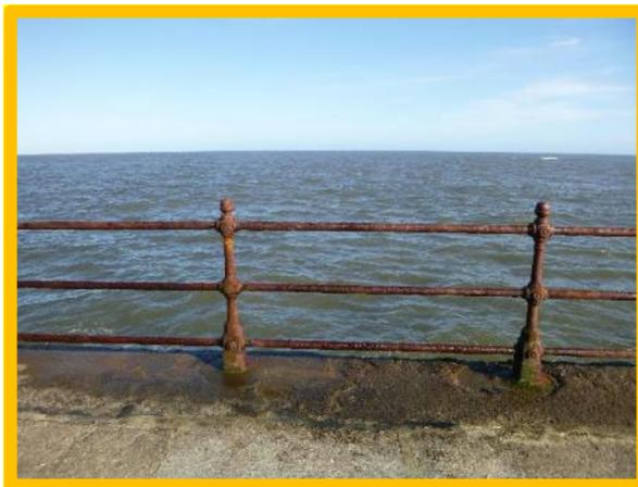
*Heavily corroded handrail (/1201C03)*
