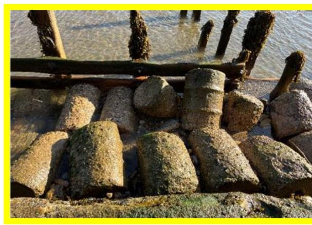
Displacement of some parts of the toe structure (D0702C01)
