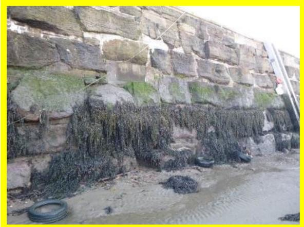
*Open joints at base of wall, principal blockwork appears in fair condition (/1301C16)*
