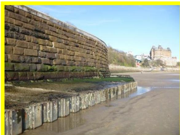
*Masonry sea wall with exposed piles at The Spa access steps in fair overall condition (/1301C27)*
