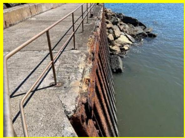
*Significant corrosion / loss of section of sheet piles (/0402C01).*
