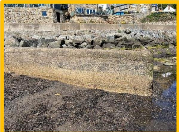
*Significant abrasion of concrete. Opening of joint between wall and crest concrete – largely obscured by vegetation (/0601C02)*
