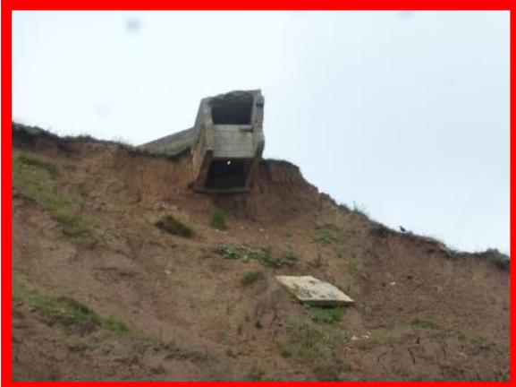
Looking from up from the beach at the base of **MU24/M1** in September 2018, note undercutting of Pill Box.
