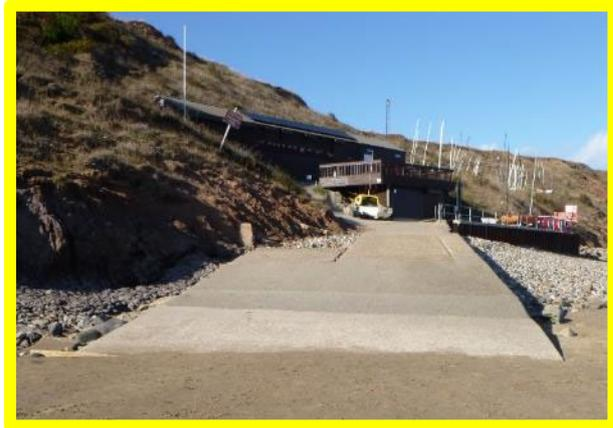
Some localised slumping of soft till onto upper section of slipway (/1601C03)
