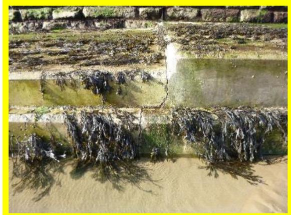
*Crack along joint in concrete apron (/1301C28)*
