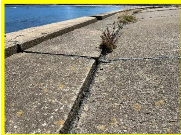
*Loss / wash-out of mortar beneath coping. Local abrasion (/0601C01)*
