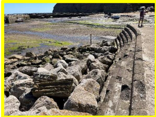
*Lower crest level at northern extent of rock revetment (/0402C02)      Southern extent of rock revetment (/0402C02)*
