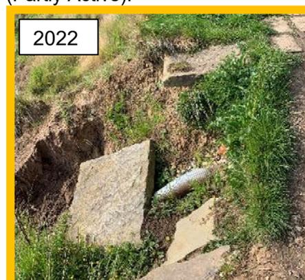
MU17/2 Undermined Cleveland Way with exposed land drainage (Partly Active).
