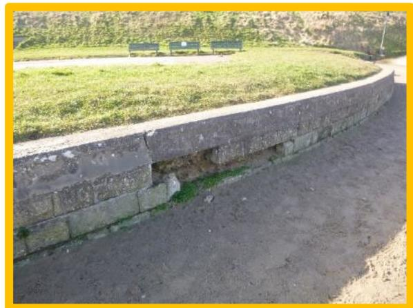
Missing blockwork in rear wall (/1201C04)
