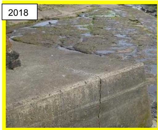
*Typical defects (cracking) on toe apron (/1003C06)*
