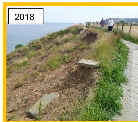
MU17/2 Undermined Cleveland Way footpath route and temporary diversion (Partly Active).
