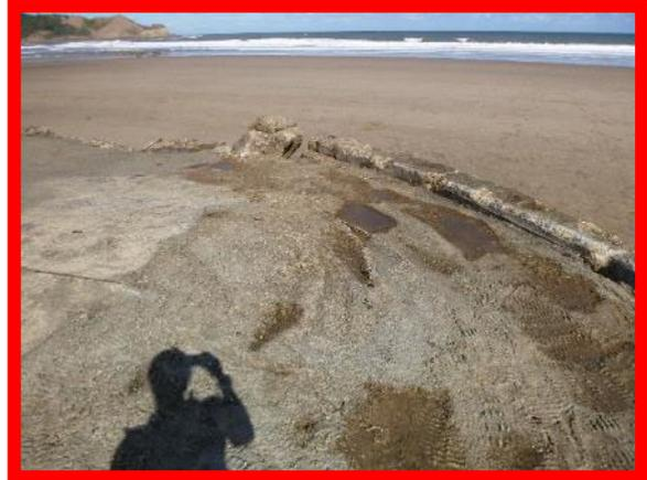
Concrete skim repair to deck slab in poor condition (/1402C04)
