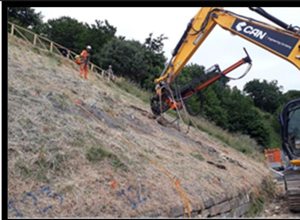
**MU22/2** Soil nail installation on coastal slopes near the Spa in 2018
