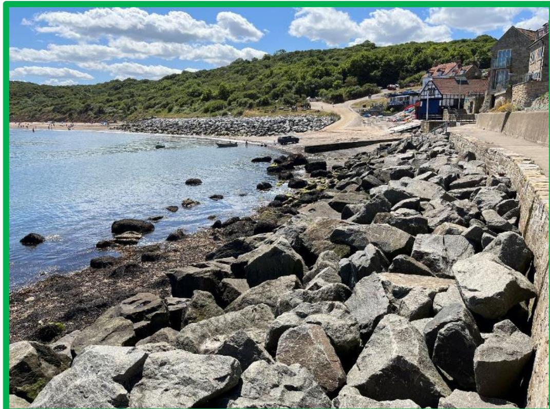
*Rock armour fillet at toe of existing seawall, seed rocks seaward of toe as constructed, July 2022.1*
