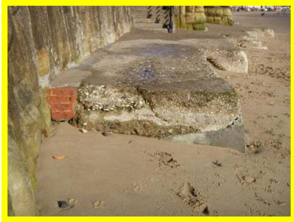
*Abrasion of toe apron south of previous repairs beach levels notably higher than 2018 (/1301C09)*
