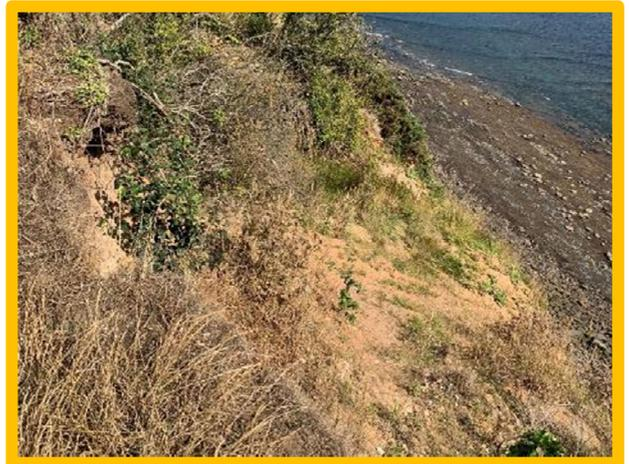
Local Slumping at MU15/3 (Partly Active)
