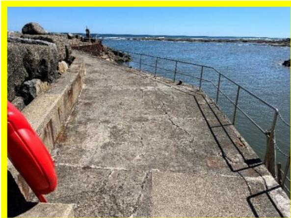
*Cracking and abrasion in deck and crest wall (/0402C01).*
