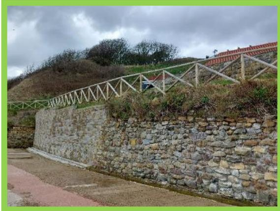
MU22/4 - recently completed retaining wall (left) transitioning into repointed pre-existing masonry retaining wall (right)
