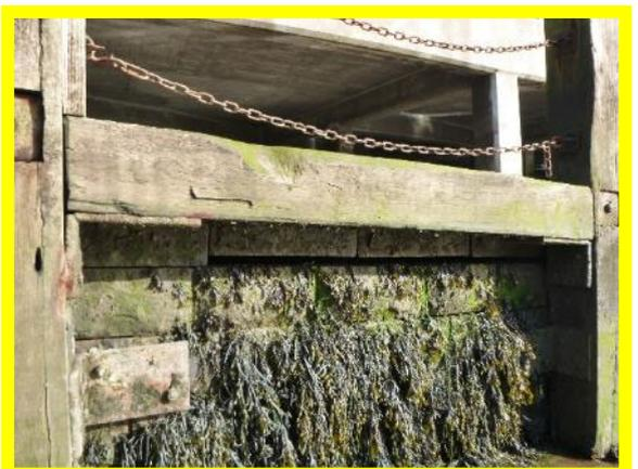
*Minor damage and displacement to blockwork wall (/1301C14)*
