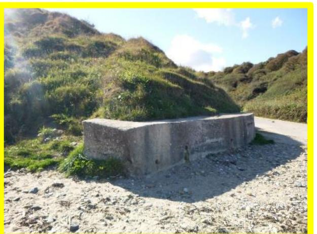
Low concrete retaining at toe of **MU29/AJ**. Evidence of localised slumping at rear of wall.
