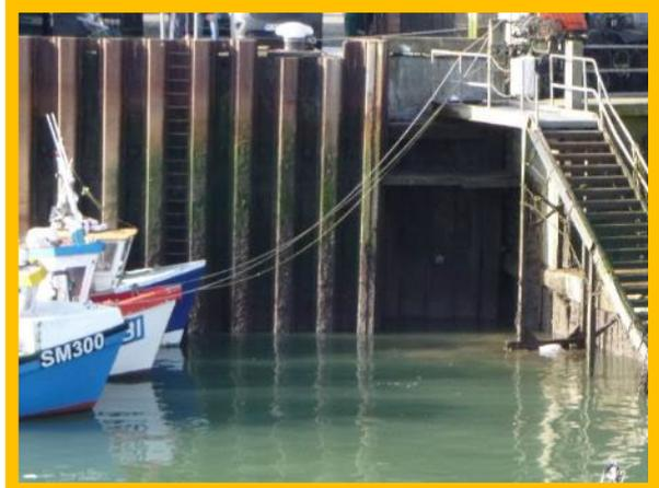
*Corroded steel sheet piling notably worse directly adjacent slipway (/1301C13)*
