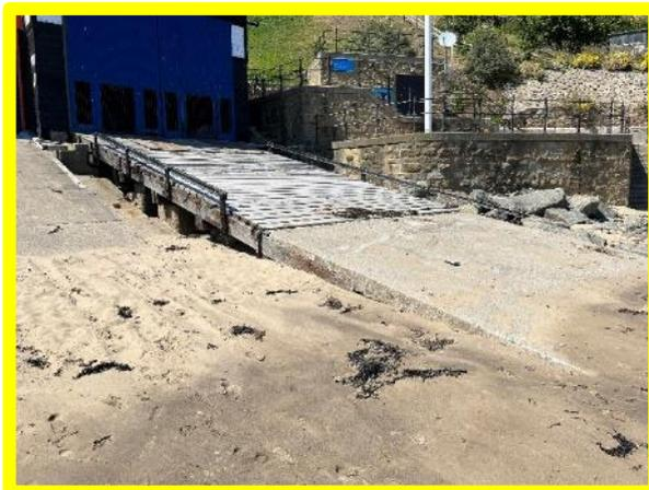
*Former lifeboat slipway. Beach levels and seaweed largely obscure previous repairs/concrete pours at the toe (/1003C04)*
