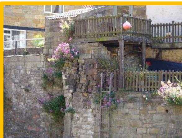
*Open joints and loose masonry blocks locally (/0402C04)*
