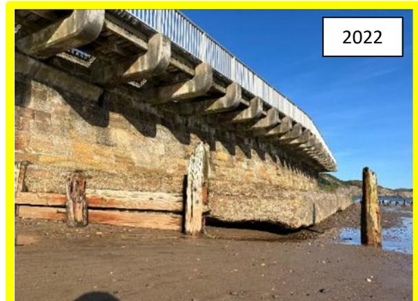
Toe structure undercut below masonry blockwork sea wall with cantilevered footway (D0702C04)
