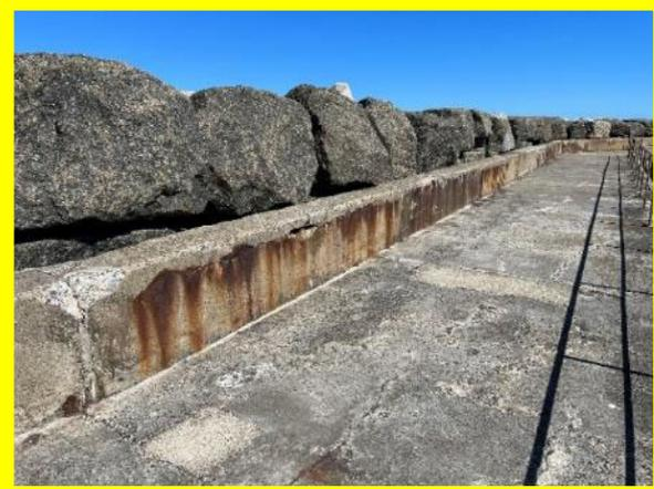
*Crack, abrasion and rust staining of crest wall (/0402C01). No significant change from 2020.*
