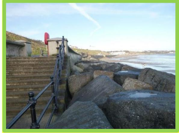
*Rock revetment fronting seawall remains in good condition (/1202C01)*
