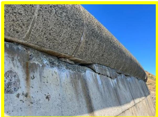
*Abrasion and cracking of concrete coping (/0601C01)*
