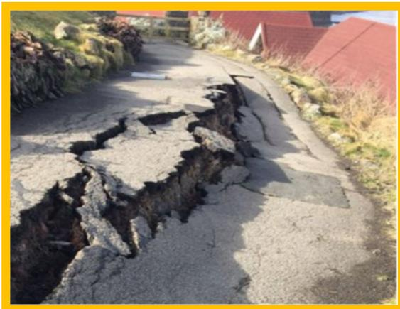
*MU22/4 large cracks in footpath above chalets in the location of the wall failure (Photo from 2018 Report).*
