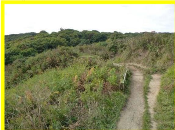
Headscarp recession has encroached on footpath. Note temporary boards to stabilise and mark path edge **MU23/F**.
