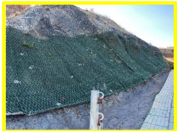
Slope protection netting above the access ramp (D0803C05)
